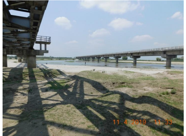
Two concrete bridge construction (Duraghati)
