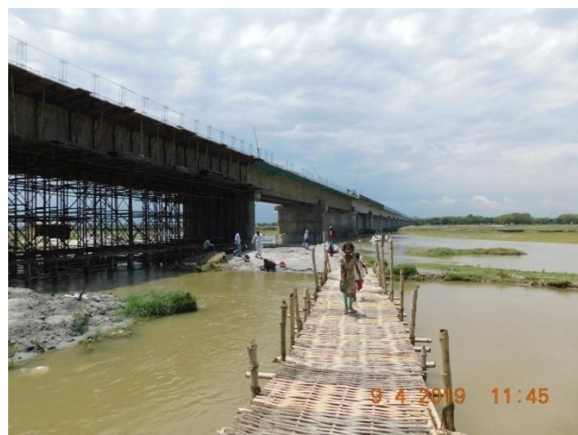
Concrete bridge construction (Loucha Ghat)
